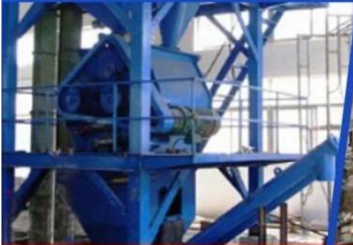
Waste incineration plant
